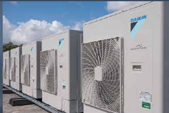
Daikin 'Seasonal Classic' roof-mounted units
