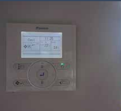
Daikin SkyAir controls
