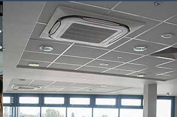
Ceiling mounted Roundflow cassette
